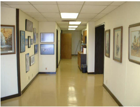
Freecom offices after removal of carpet, preparation of concrete, application of CeRam-Floor Slurry (do to concrete being very uneven), topcoat with CeRam-Kote 99M. Walls and trim painted with CeRam-Thane 100. Star Design by Freecom
