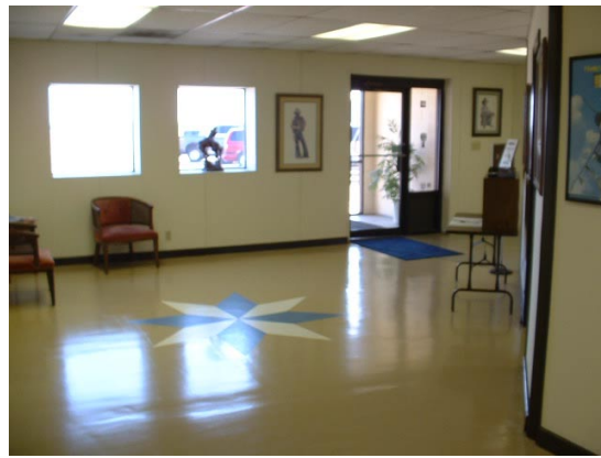
Freecom offices after removal of carpet, preparation of concrete, application of CeRam-Floor Slurry (do to concrete being very uneven), topcoat with CeRam-Kote 99M. Walls and trim painted with CeRam-Thane 100. Star Design by Freecom
