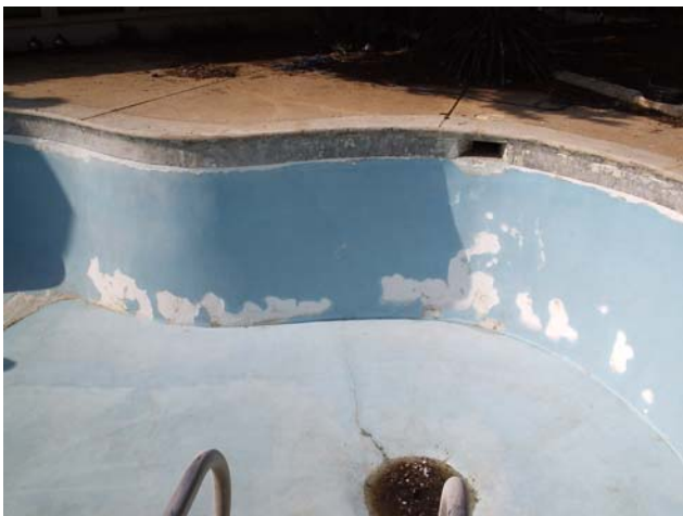
Preparation included vacuum, high-pressure water blast, and degreasing several times
