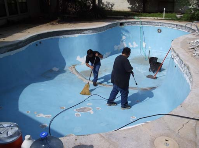
High-pressure water cleaning with tri-sodium phosphate detergent.
