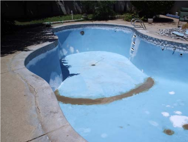
Refurbishing grout material to repair large crack and holes
