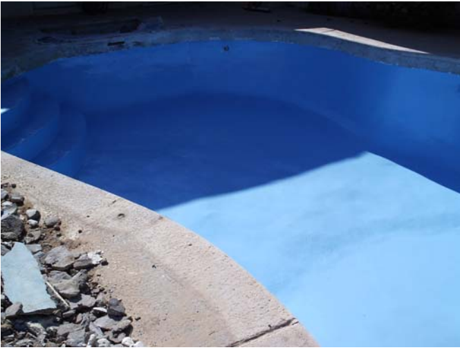
CeRam-Kote 99P Blue applied in three passes
