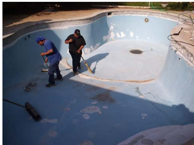
Preparation included vacuum, high-pressure water blast, and degreasing several times
