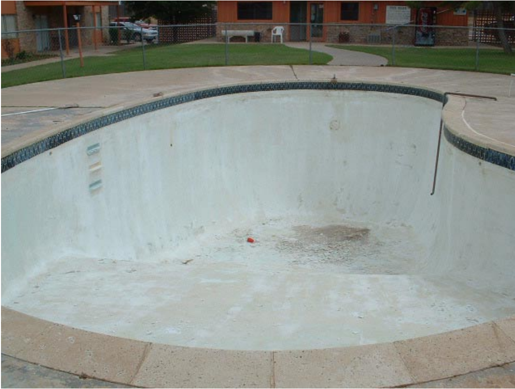
Ponderosa Pool #2: Before preparation and application March 2003
