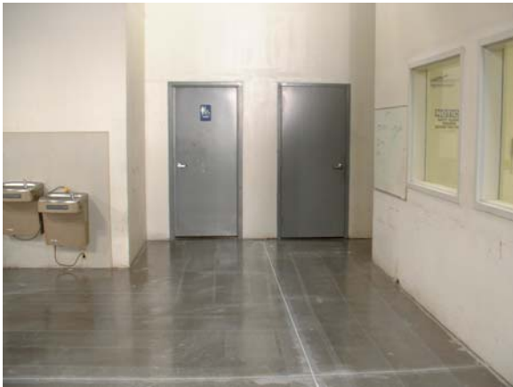
CeRam-Floor Primer was applied over entire blasted surface. Average thickness = 4 mils (100 microns).
