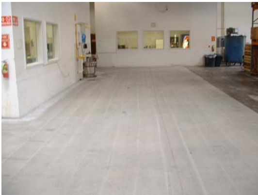
Floor was prepped via steel grit using a USF-Blastrac unit.
