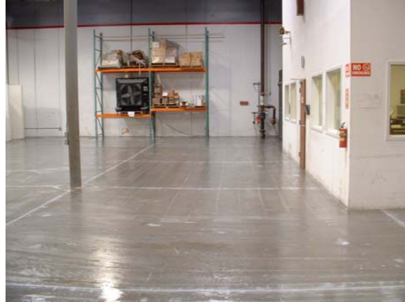
CeRam-Floor Primer was applied over entire blasted surface. Average thickness = 4 mils (100 microns).
