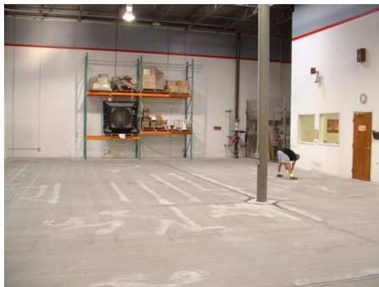
All saw cut areas were filled with CeRam-Floor filler
