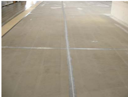
All saw cut areas were filled with CeRam-Floor filler
