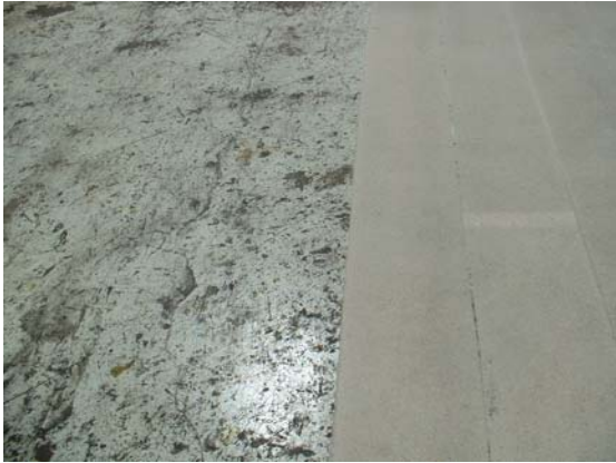
Floor was prepped via steel grit using a USF-Blastrac unit.
