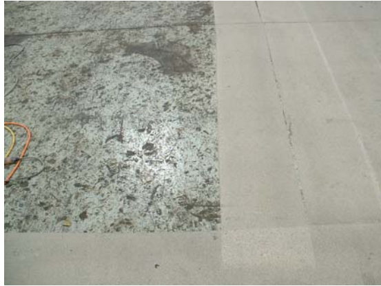
Floor was prepped via steel grit using a USF-Blastrac unit.
