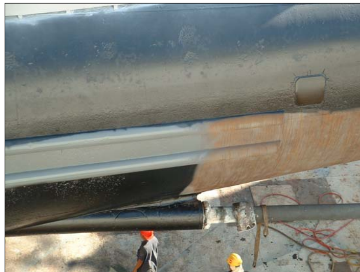
CeRam-Kote SPG applied over primer coat of CeRam-Kote 99M
